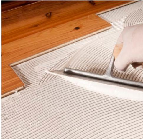
EFA+™ Elastomeric Flooring Adhesive is a one-part, trowel applied, moisture-cure urethane adhesive; this adhesive does NOT contain any water. Once cured, EFA+ is waterproof and is not adversely affected by exposure to moisture or water. When applied as directed for a moisture vapor membrane, EFA+ will reduce moderate amounts of moisture vapor transmission from the subfloor and prevent damages to engineered wood flooring caused by subfloor moisture.
